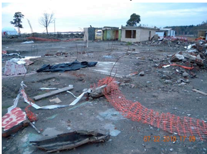
Figure 12. Earthquake and tsunami damage in the coastal city of Constitución.
