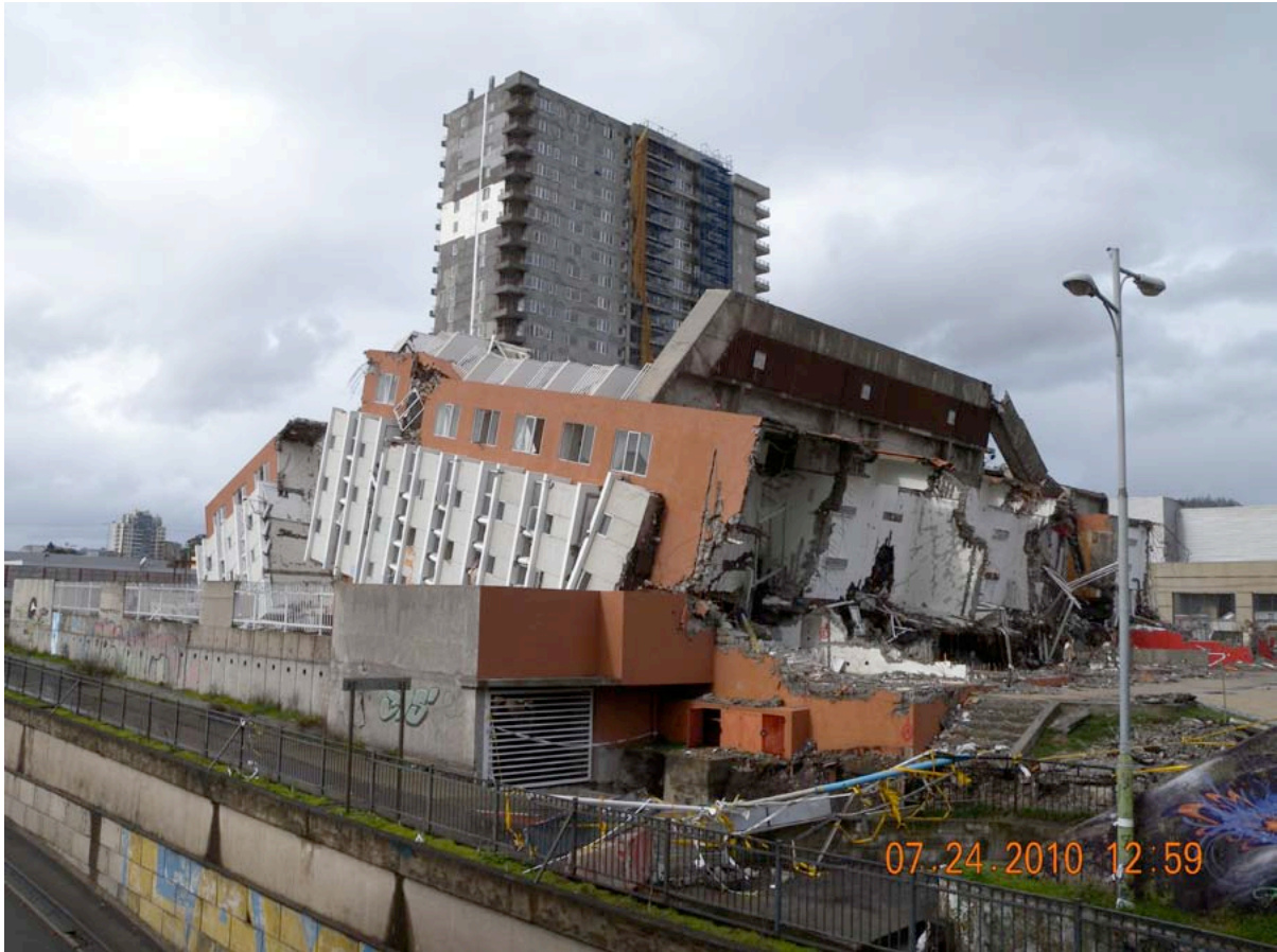
Figure 4. The collapsed Alto Rio apartment building in Concepción. Eight people were killed when this building fell over.
