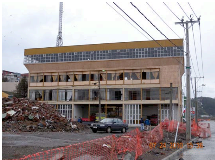
Figure 8. Damaged Firehouse in Talcahuano, near Concepción.
